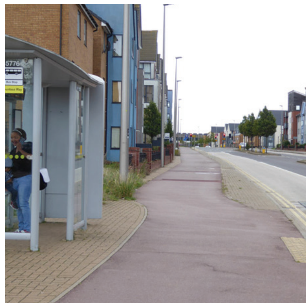
Figure 19: A coherent street suitable for bus operation, with planted median and frontage development. The design also includes bus lanes and bus-friendly traffic calming (Milton Keynes eastern expansion area). (Photo: Tim Pharoah, 2017)
