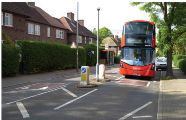
Figure 30: Correct speed cushion placement (Dover House Road, London) (Photo: Tim Pharoah, 2017)
