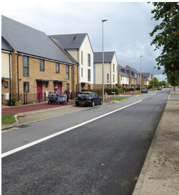
Figure 18: A coherent street suitable for bus operation, with planted median and frontage development (Broughton, Milton Keynes) (Photo: Tim Pharoah, 2017)
