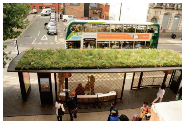
Figure 37: 'Concept shelter' with screen in centre of footway arranged to provide shelter on either side. Note also the green roof. (Photo courtesy of Transport for Greater Manchester)
